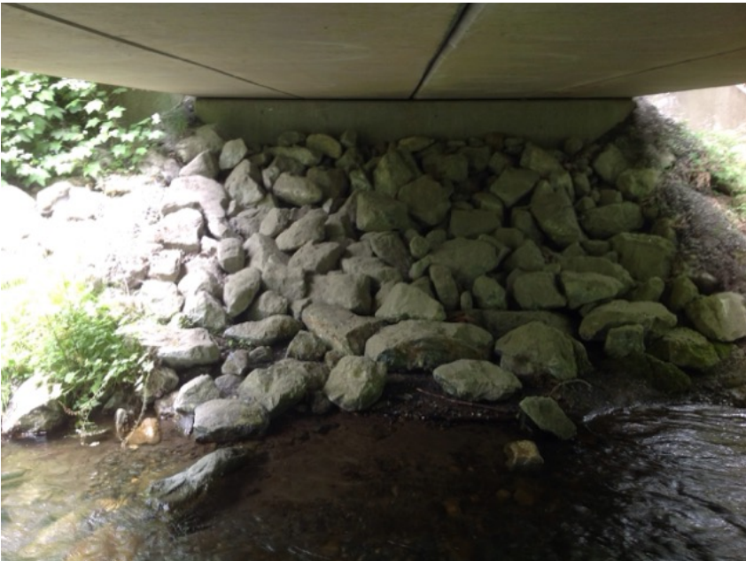
Left Bank Abutment when facing downstream
