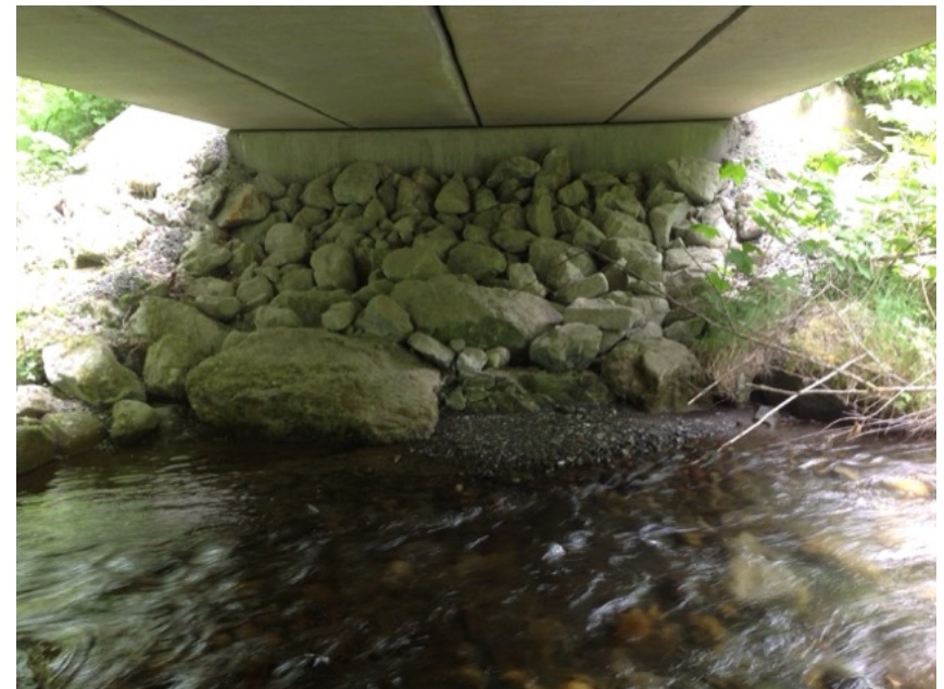
Right Bank Abutment when facing downstream
